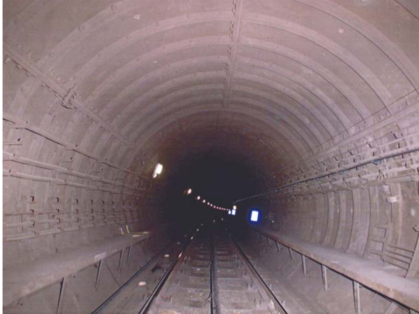
Fig 1 - Photograph of typical tunnel section
