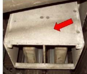
Figure A Cement panel boxing 1.8m 2 To arc chute, Chrysotile
