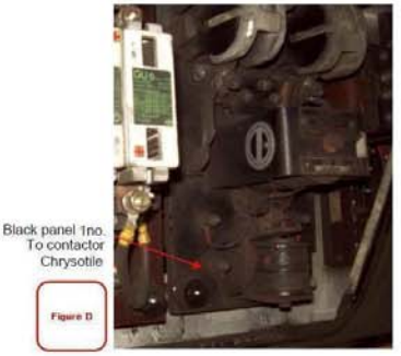
Figure D Arc chutes 2no. To contactor Chrysotile
