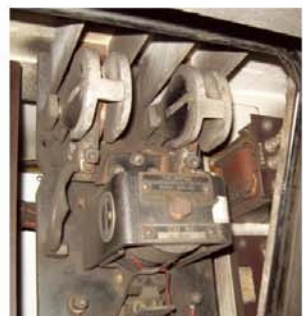
Figure D Arc chutes 2no. To contactor Chrysotile
