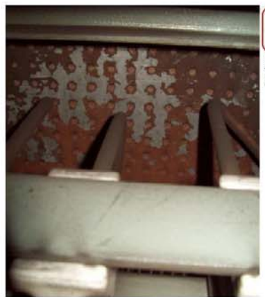
Figure F Durasteel 10m 2 To mid section above resistor grids A, B and C Amosite & Chrysotile
