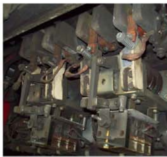
Figure E 2no. <1m 2 Cement Panel To switch behind large arc chutes Chrysotile
