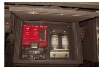
Figure B Cement panels / lining 0.25m 2 Within main negative fuse box Chrysotile
