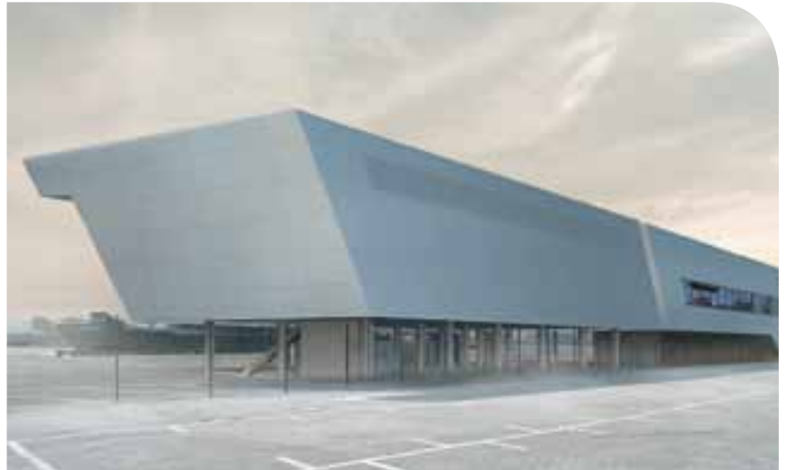
OPS infrastructure at cruise terminal Hamburg-Altona
