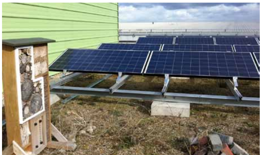
Photovoltaic panels, combined with a living roof and a 'bug hotel' on the Olympic Park
