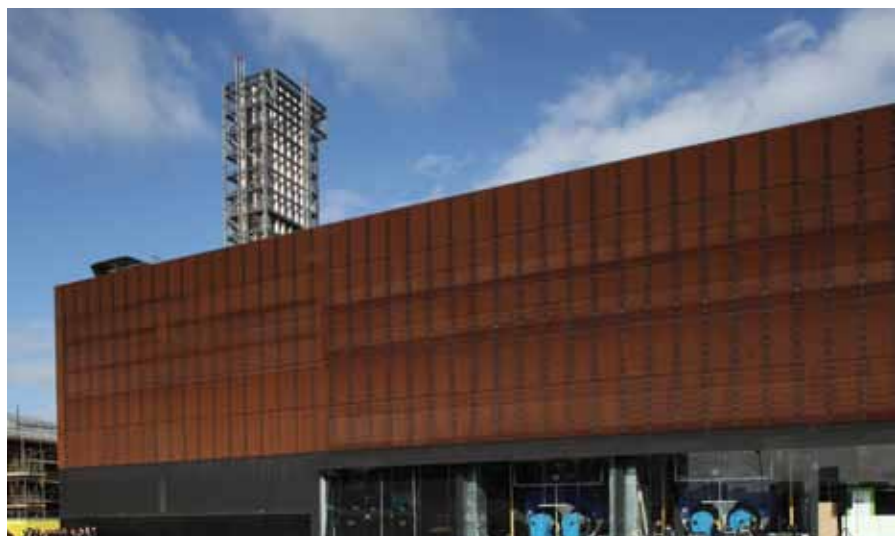
The Energy Centre on the Olympic Park
