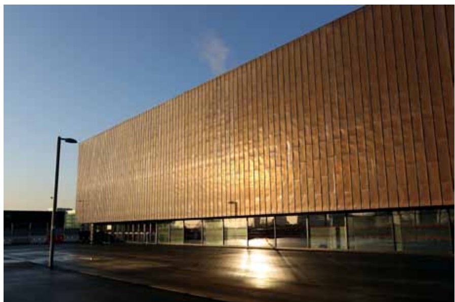
The Eton Manor sports complex is the only timber frame building on the Olympic Park, constructed of glulam beams
