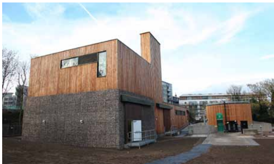
Old Ford Water Recycling Plant
