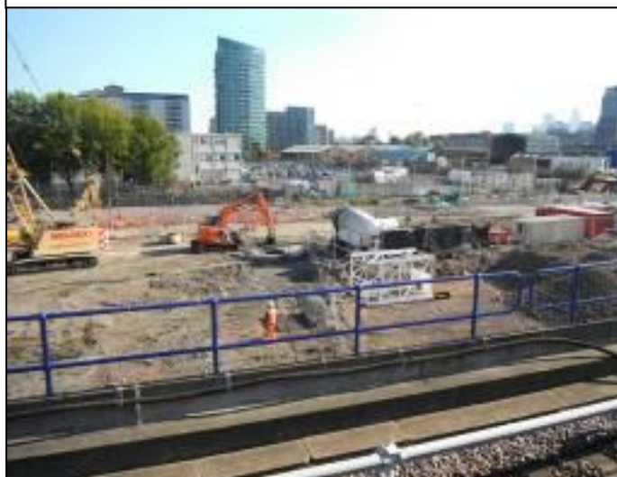
Figure 6.4: Crossrail Site at Pudding Mill Lane
