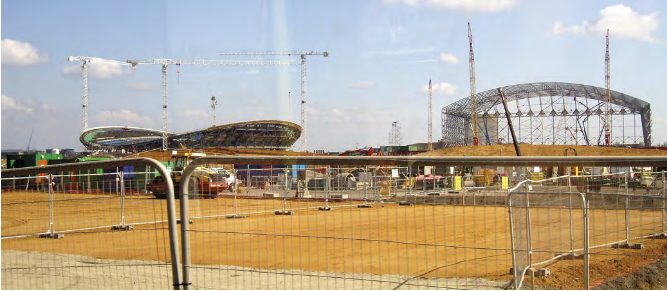
Olympic Park under construction.
