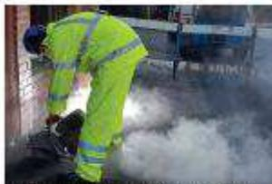
Figure 1. Common tasks like cutting can create very high dust levels.
